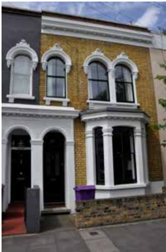
Strahan Road (with original cornice intact).
