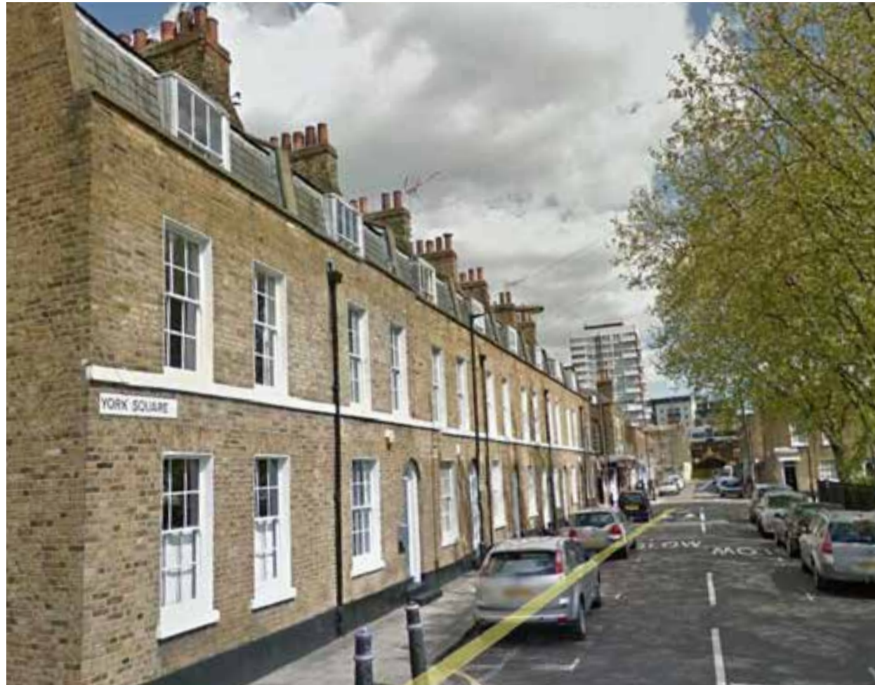
A unified approach to design was adopted when mansard roof extensions were added to York Square E14
