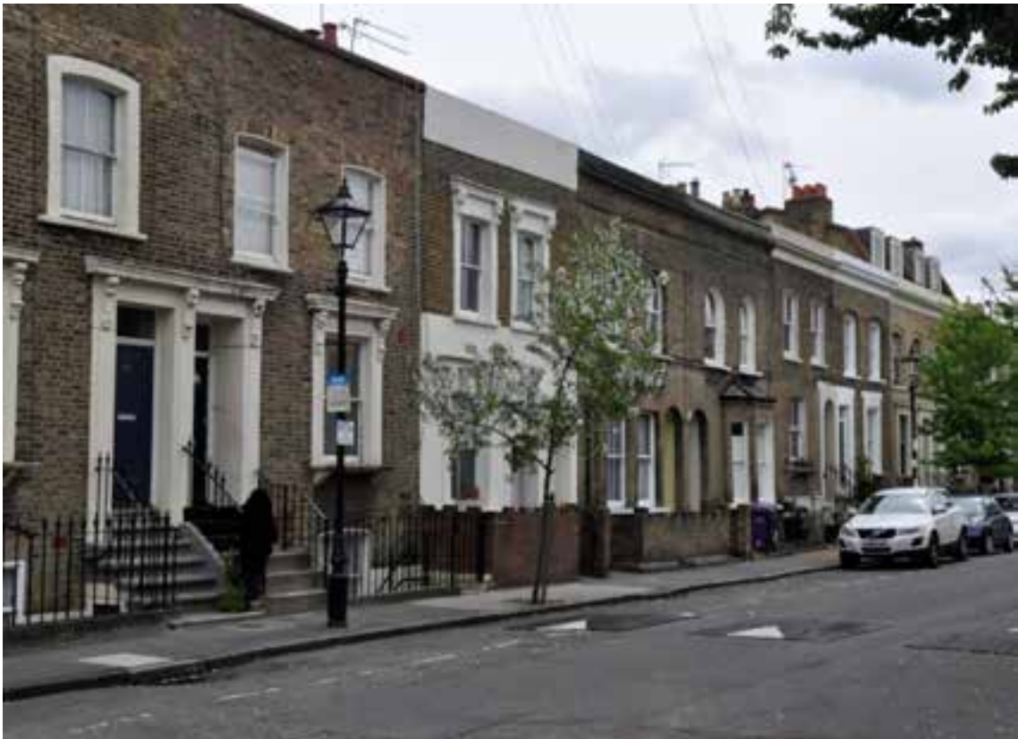
Kenilworth Road. Some houses have steps above semi-basements while others in the street do not.
