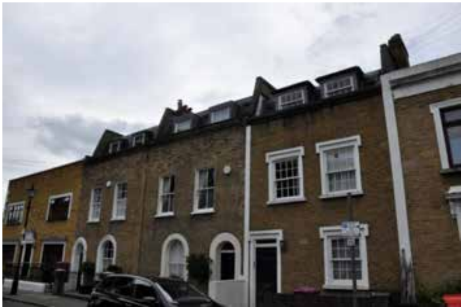
Existing mansard roof extensions on Norman Grove.
