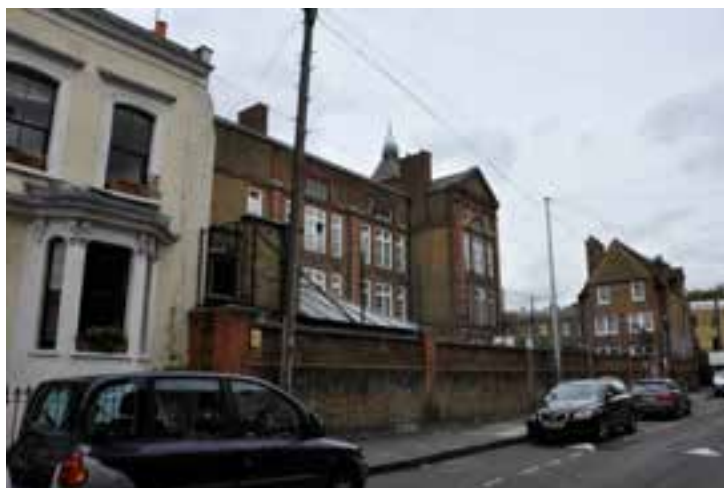
View of Chisenhale Primary School from top of Zealand Road.
