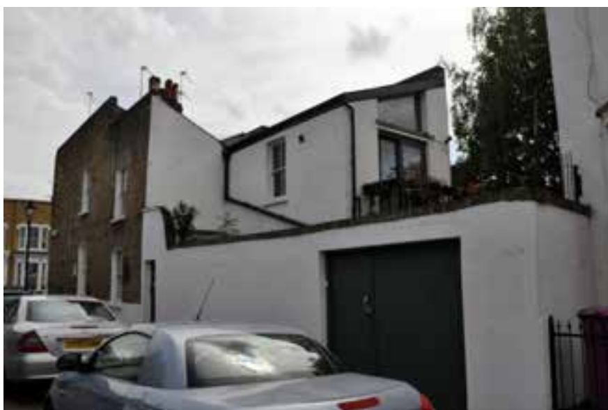
Rear extension along Medway Road.
