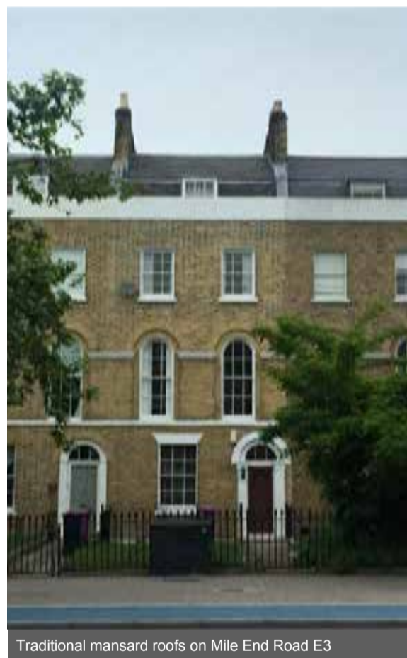
Traditional mansard roofs on the corner of Mile End Road and Tredegar Square E3
