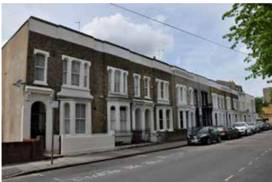
Terrace on Selwyn Road; the houses have canted bay windows but only three houses retain their cornice.
