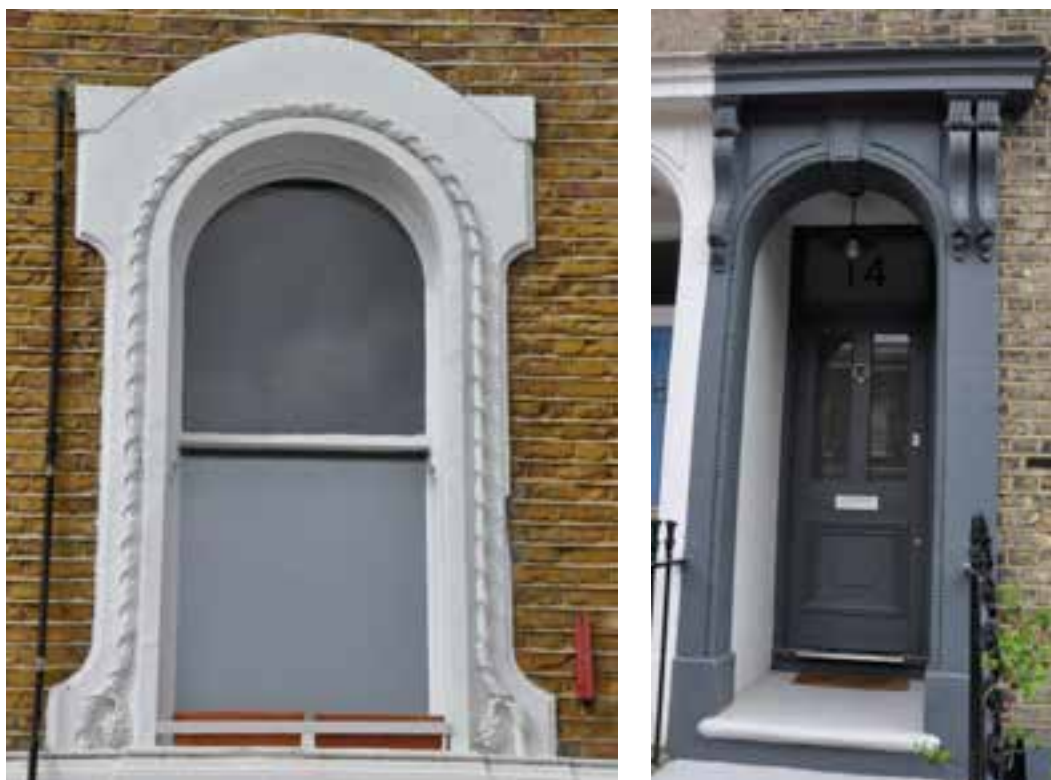
Rope mouldings (of various styles) decorate the architraves of windows and doors, seen here in Hewlett Road (left) and Ellesmere Road (right). This detail can also be seen in the window architraves of some properties in both Kenilworth Road and Vivian Road.
