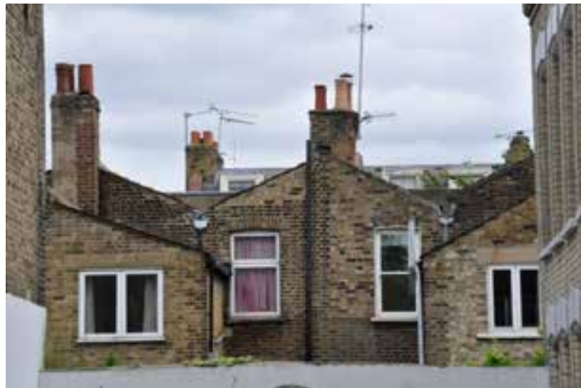
The rear elevation of the butterfly roofs of properties on Kenilworth Road, as seen from Grove Road. Note also the pairs of chimney stacks located along the party walls.
