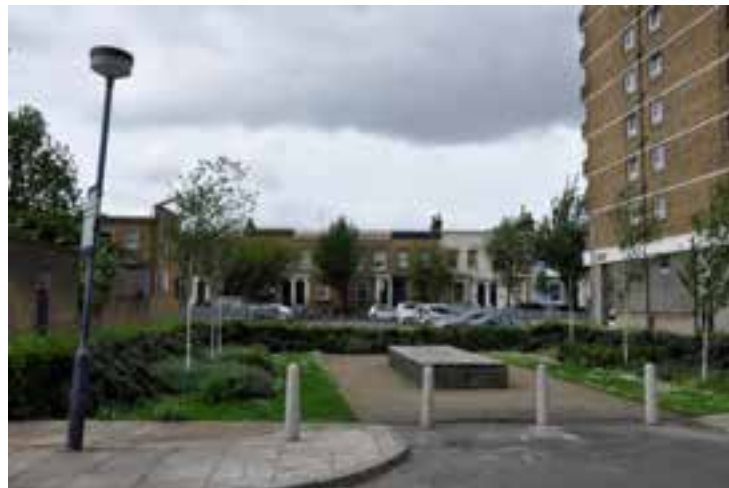
View from Hewlett Road to Driffield Road: consistent parapet height.
