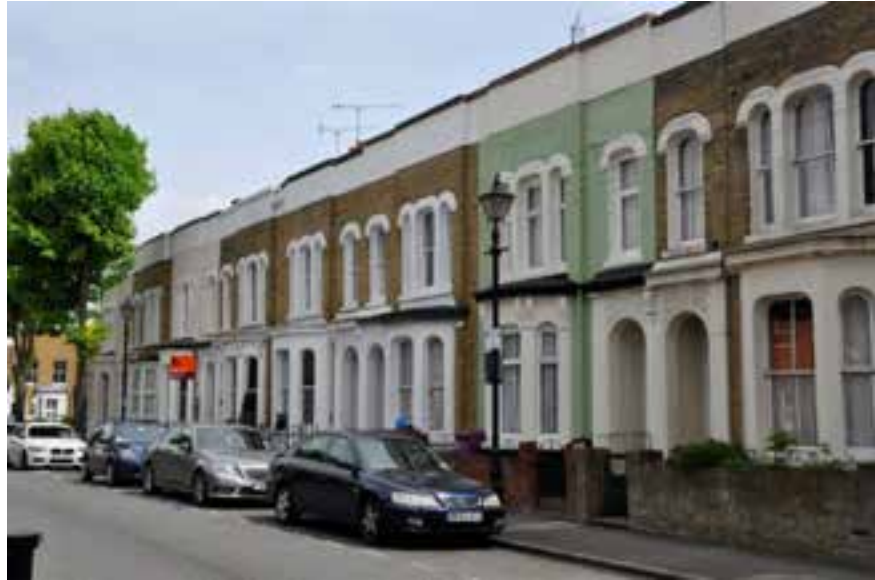
Antill Road. This photograph shows the alternating recess to the front elevations, some of which have been painted, and all in this image are missing their original cornices.
