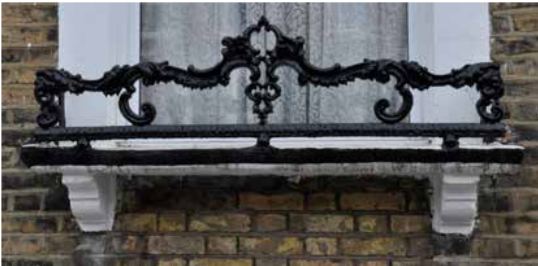
Different types of wrought ironwork window guards. Both of the above examples are from Driffield Road but these guards are also present on some properties in Ellesmere and Vivian Road.
